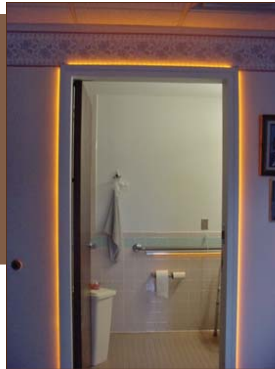
(Figure 9a) Delineation of transitions zones. Horizontal and vertical lighting provides perceptual cues to help older adults orient themselves when awaking from sleep. These amber LEDs are photosensor and motion controlled. Amber was selected because it gives enough light to see and is closest in color to the familiar incandescent.
